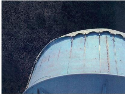
Figure 4: Missing Radome Mounts
