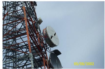
Figure 3: Heavily Damaged Radome
