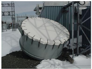
Figure 1: Microwave Antenna with Radome
