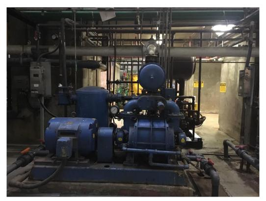
Figure 2: Unit 2 Vacuum Pump
