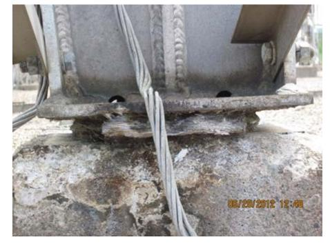
byproducts between the baseplate and the surface of the concrete foundation (Figure 1).
