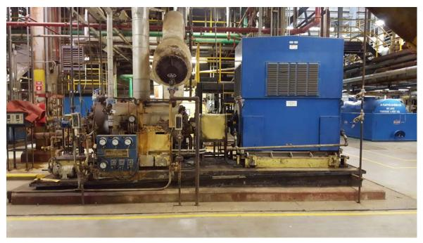
Figure 1: Unit 2 Boiler Feed Pump
